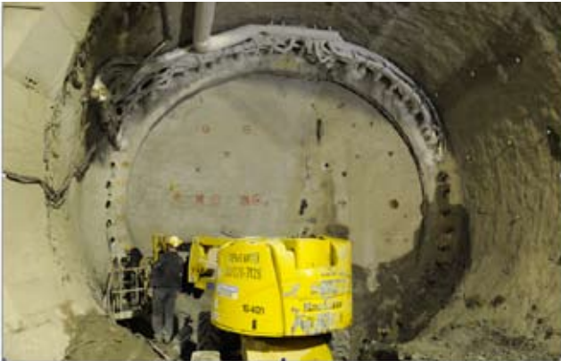
6. Figure: Ground freezing pipes under the Danube on the Fővám station
