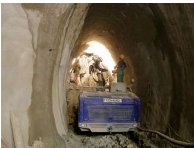
7. Figure NATM Tunnelling- Kálvin tér station
