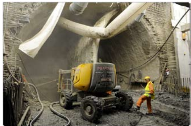
4. Figure NATM Tunnelling- Kelenföld railway station
