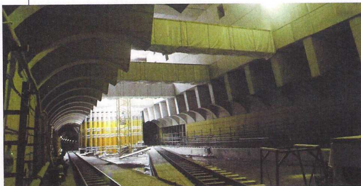
Below: Works underway at Móricz Zsigmond Square Station following TBM passage
