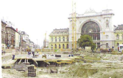
Above: Open cut station construction works underway at Bocskai road station and Keleti main railway terminus
